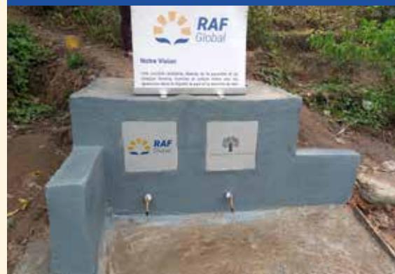
After Water Tank Construction
