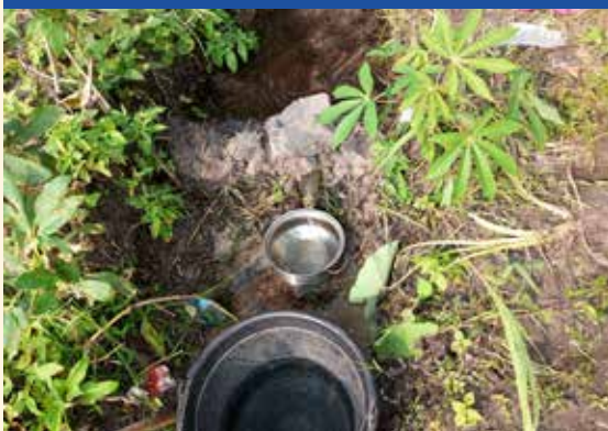
Before Water Tank Construction
