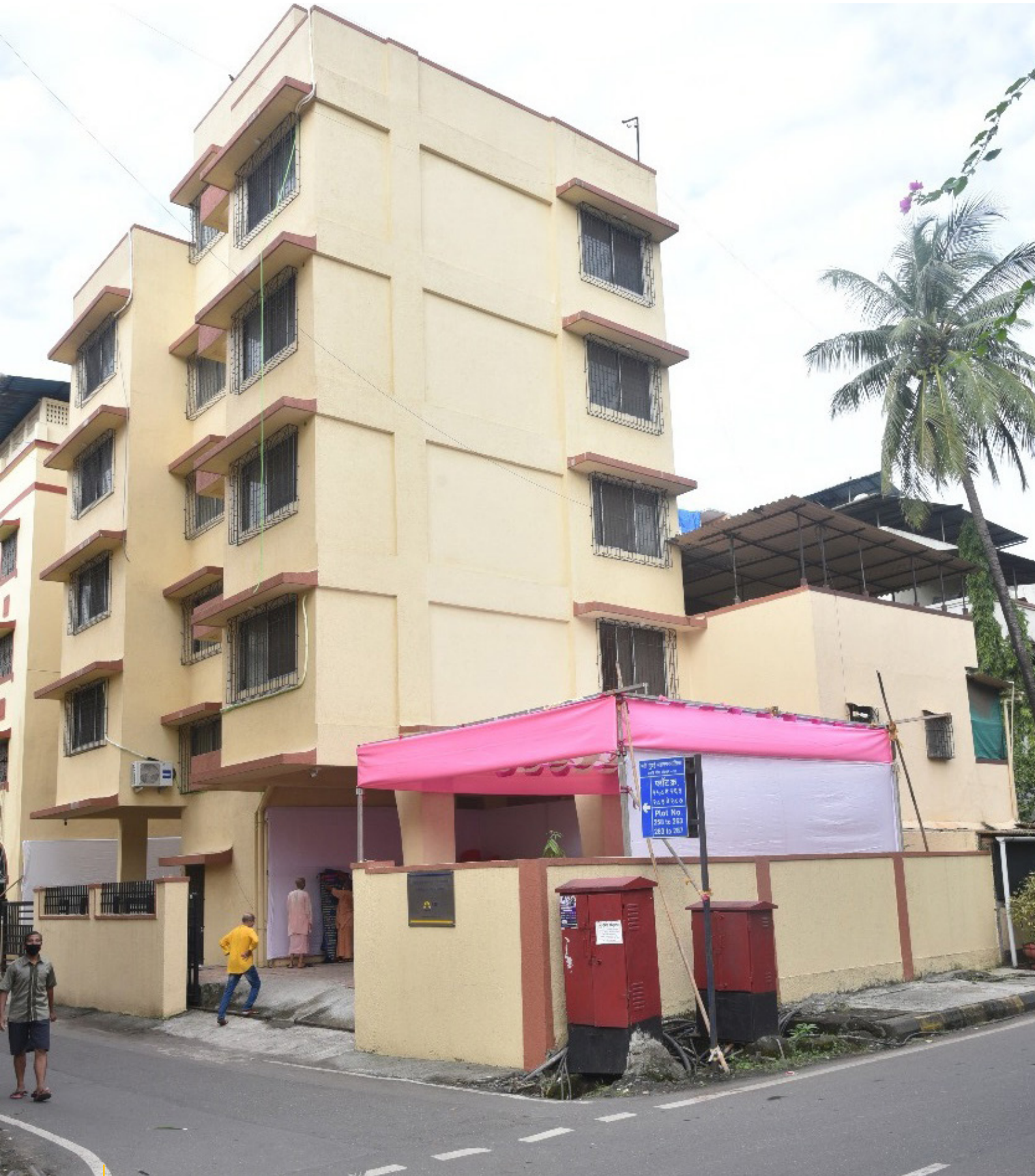
A view of RAF Global supported Cancer Facility for poor outstation patients in Navi Mumbai, Maharashtra, 2021
